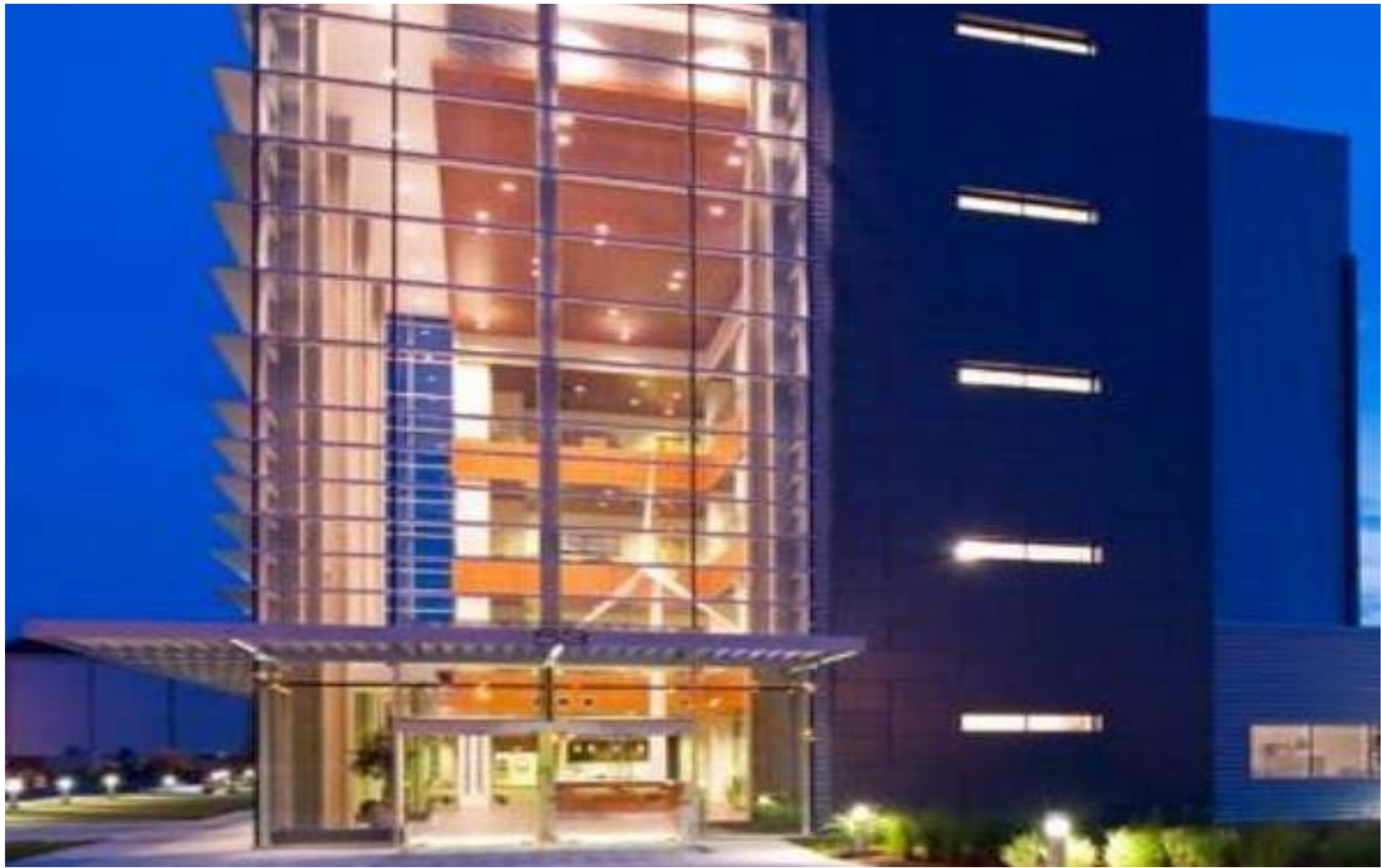
OFFICE / COMMERCIAL - Building frontage along public streets and open space will be pedestrian oriented on the first floor.
