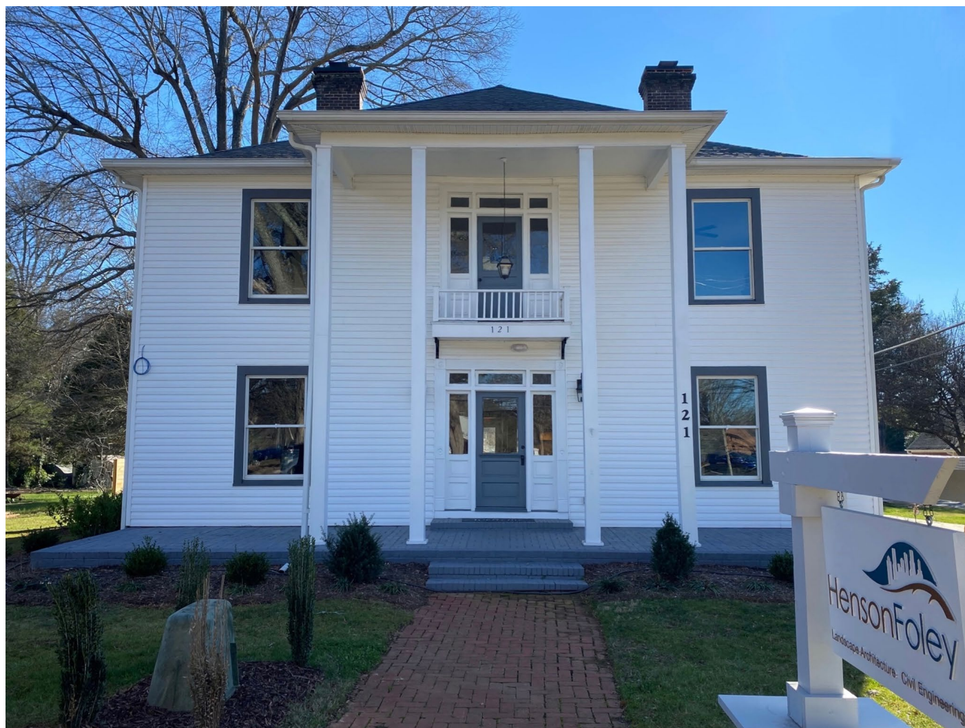
Fig. 2: Front (North) Elevation
