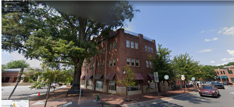
Mixed-use building with commercial 1 st floor except for residential access.
