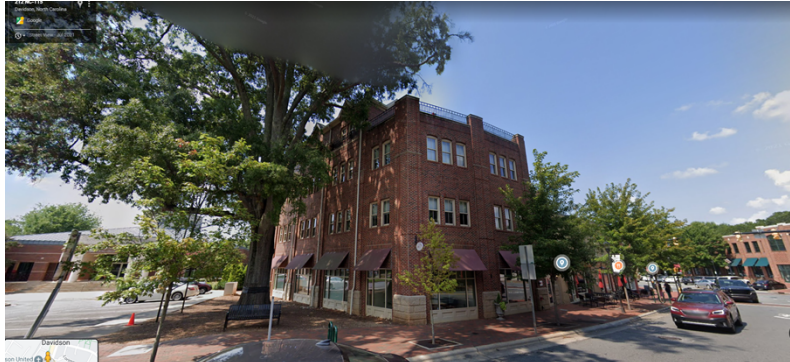
Mixed-use building with commercial 1 st floor except for residential access.
