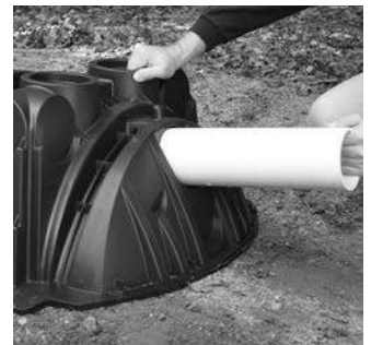
5. Insert inlet pipe.
