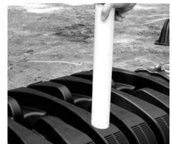
Chamber inspection port.
