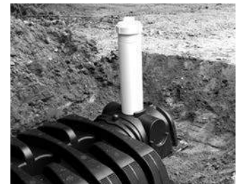
Endcap inspection port, top.
