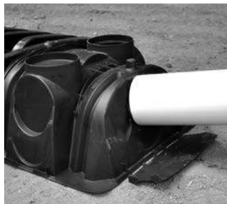
5. Insert inlet pipe.
