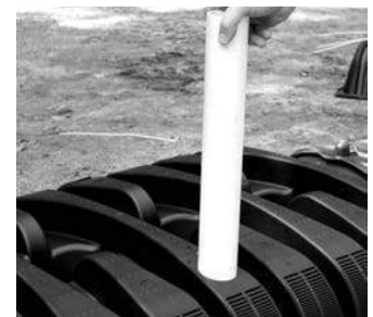
Chamber inspection port.
