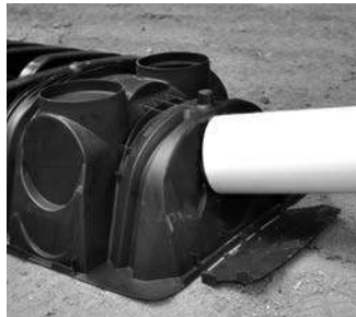
5. Insert inlet pipe.
