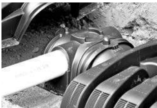
6. Insert connection pipe into endcap opening.
