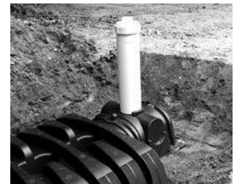
Endcap inspection port, top.
