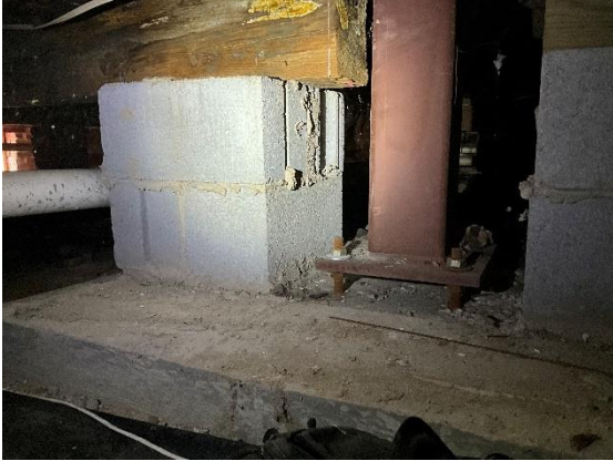
Photo 8: Provide Non-Shrink Grout
