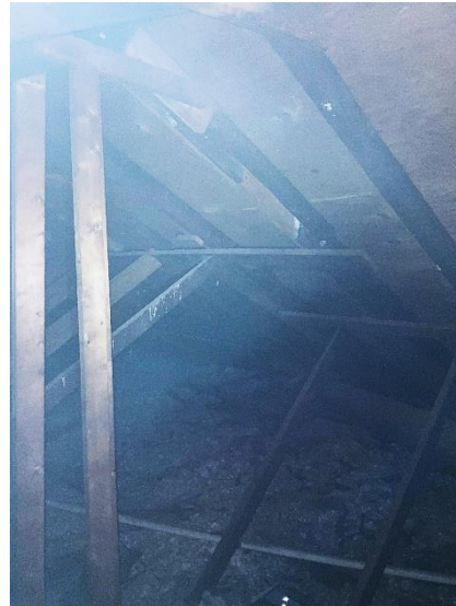
Photo 7: Typical Condition of Attic/Roofing System
