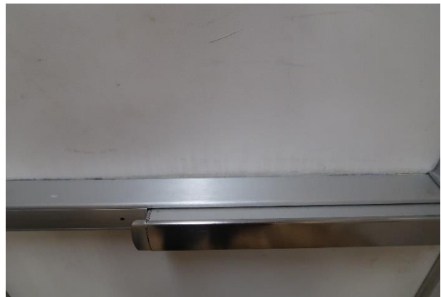
Photo 21: Evidence of Water Infiltration at Rear Entry
