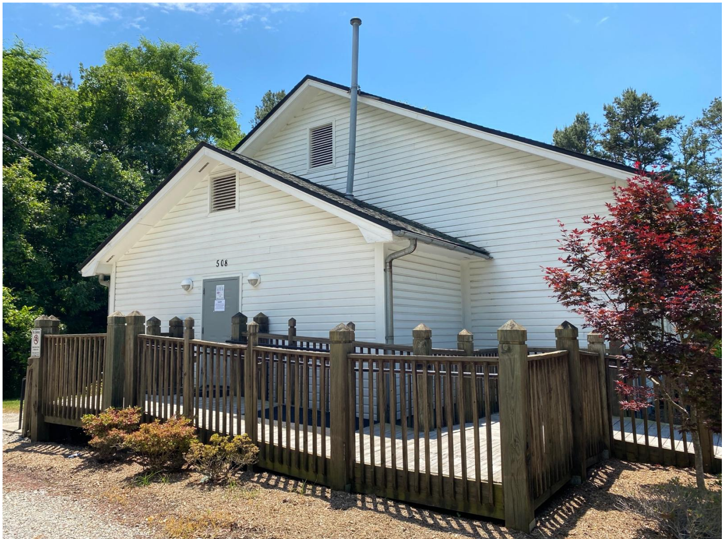
Fig. 2: Front (North) Elevation
