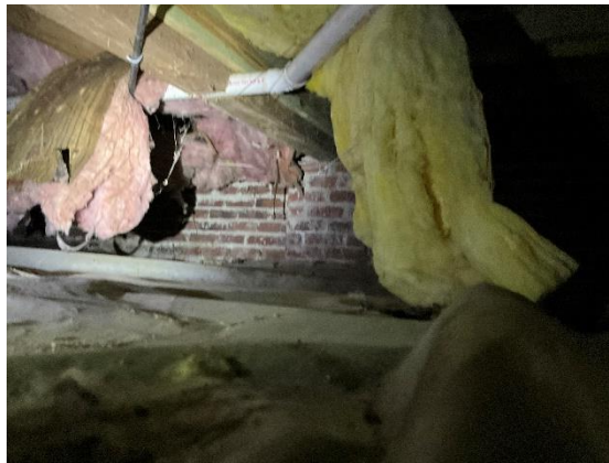
Photo 10: Reinforce 8x6 Girder Under Kitchen
