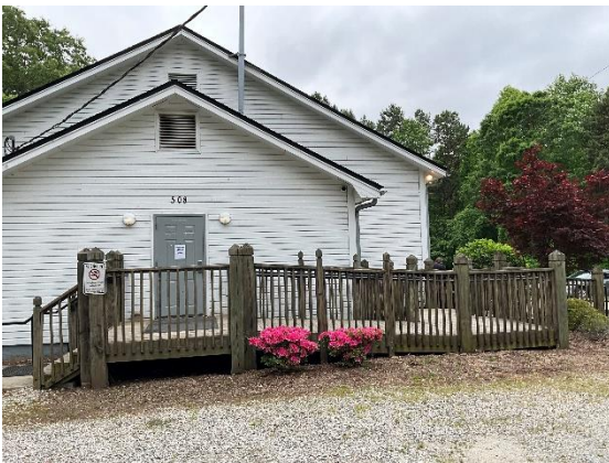
Photo 6: Front Entry Ramp
