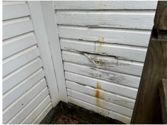
Photo 14: Deteriorated Siding
