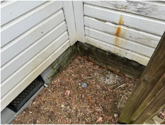
Photo 13: Deteriorated Siding
