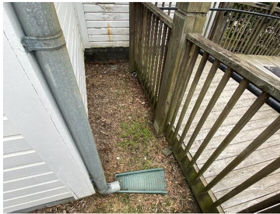
Photo 5: Install Hard Pipe and Regrade to Provide Discharge Away from Building
