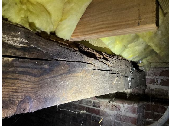
Photo 9: Replace Rotted 8x6 Girder
