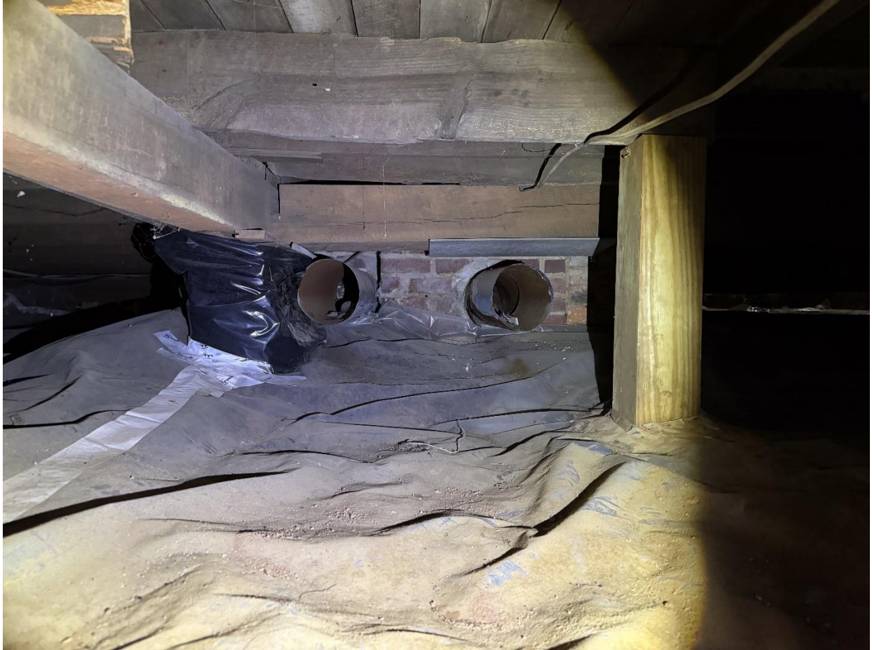
Figure 13 View at the crawlspace looking north toward the brick chimney. The wood plank subfloor at the top of the photo runs perpendicular to the floor beams, identifying this portion of the Caldwell-Bradford School as the original portion.
